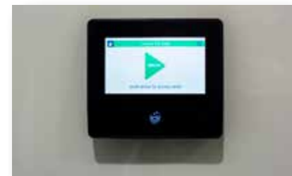
New option LCD touchscreen controller with inbuilt user tutorials and security functionality.
