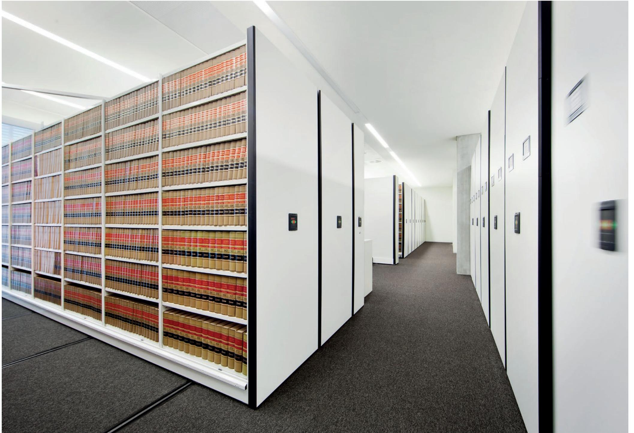
Dexion's solution involved one of the largest installations of Compactus® units in the country – a total of 19 automated Dexion Eclipse Compactus® and another seven Dexion Mechanical Assist together formed over 3,000 lineal metres of file storage.
