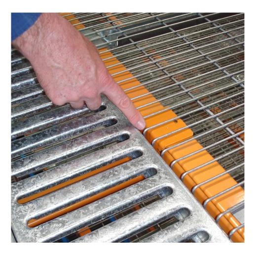
U-shaped hangers. These sit over the rack beam and support the steel grid flooring panels from below, keeping the flooring panels flush with the deck enhancing OH&S.
